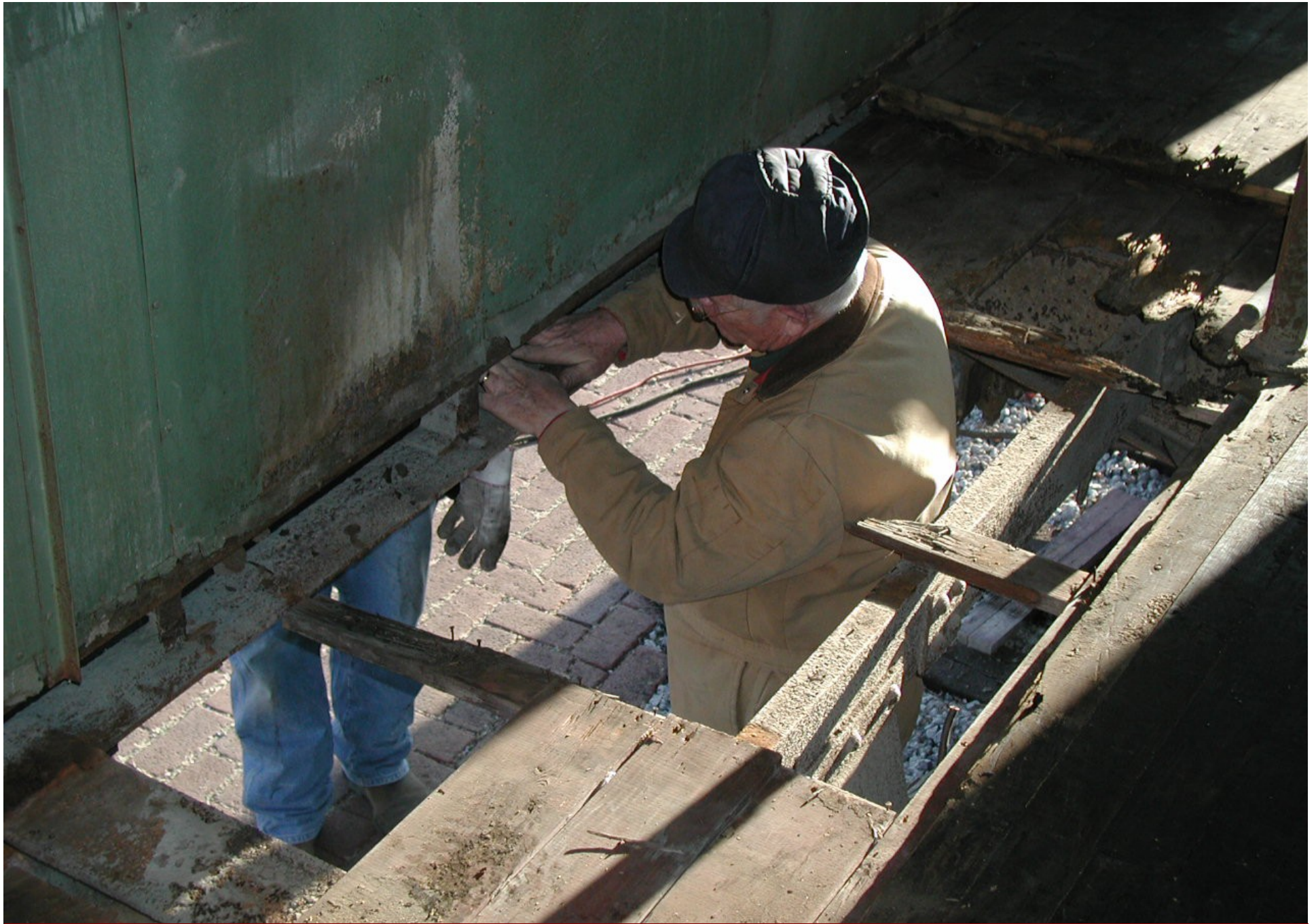
The lavatory had completely rotted a large section of the floor and subfloor.
